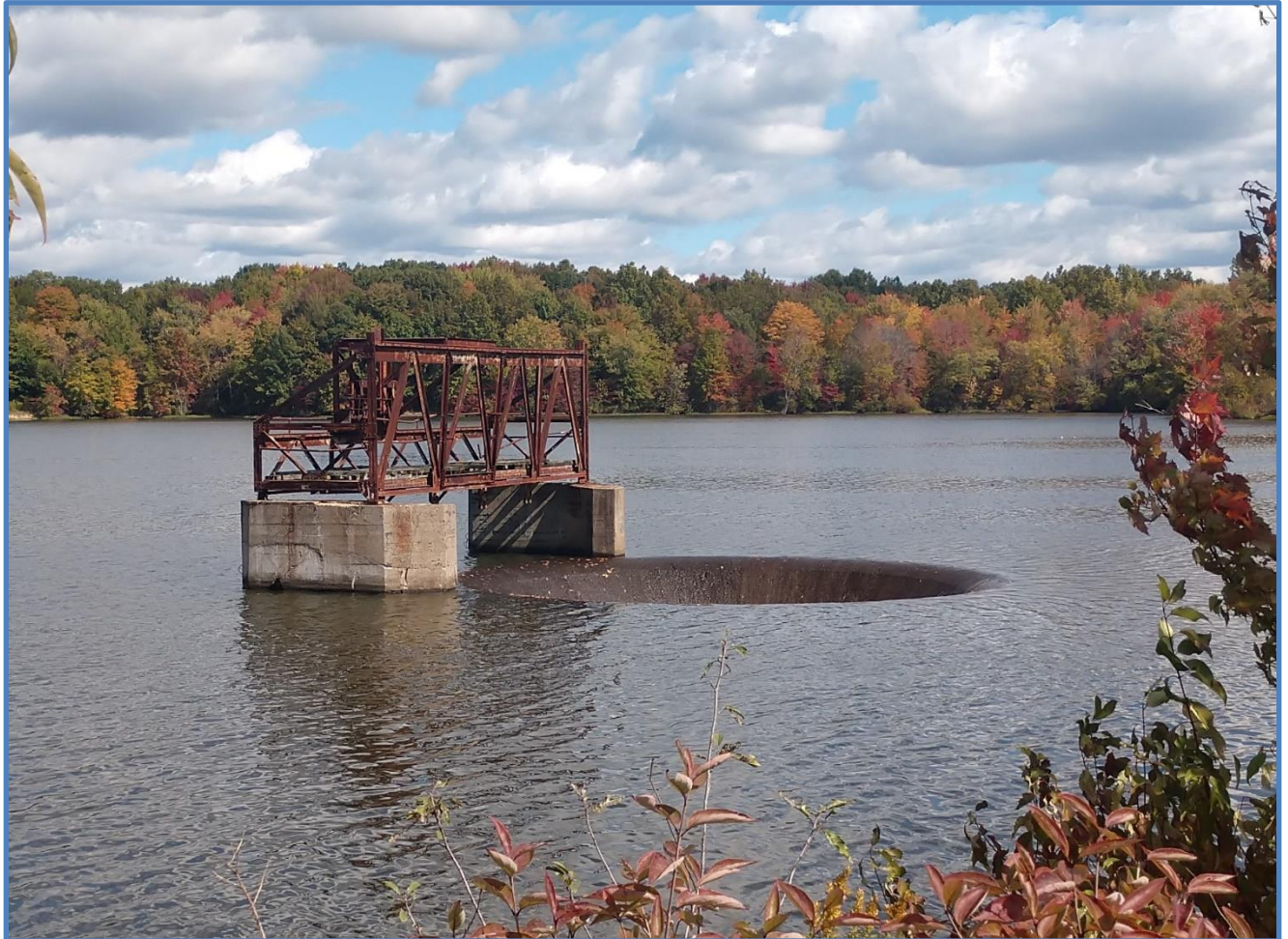
Upper Girard Lake Morning Glory Spillway
